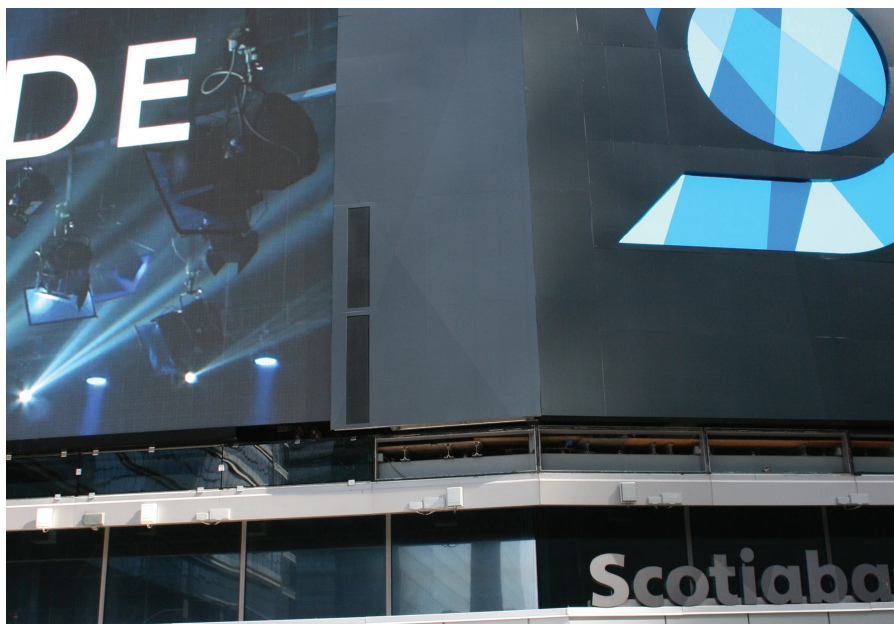
FOUR DISCREET RENKUS-HEINZ ICLIVE X MODULES COVERING THE SOUTH SIDE OF MAPLE LEAF SQUARE
